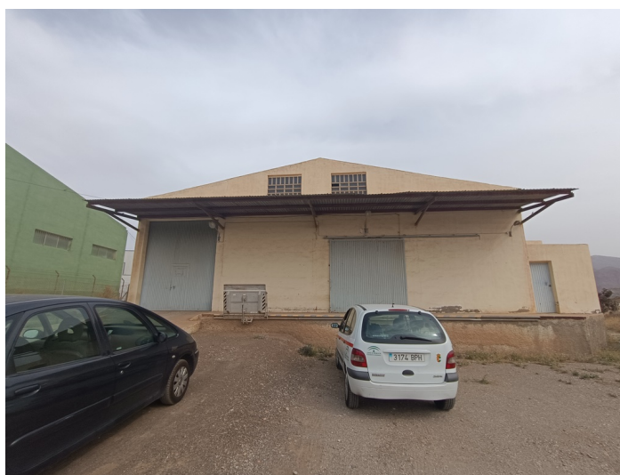
Vista Fachada Principal
